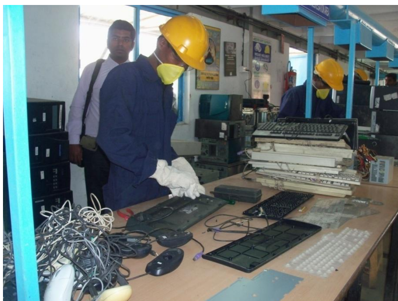
Figure 2: Dismantling being carried out by skilled workers using safety gadgets at Earth Sense Recycling Facility at Hyderabad
