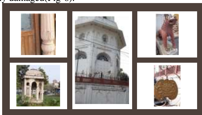
Fig-6 Safed Baradari visibly damaged.
