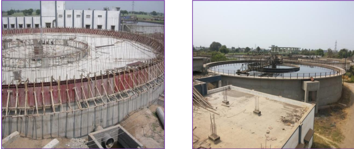
Figure 2: Ground Supported Circular Tanks of 30 metre and 42 metre diameter with Obstruction inside Tank for Effluent Treatment Plant at Surat
