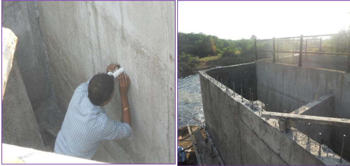
Figure 9. Crack width measurement using microscope 40-X on ground supported rectangular and circular tank at Surat near Kadoara –Ahmedabad national highway for Effluent Treatment Plant.
