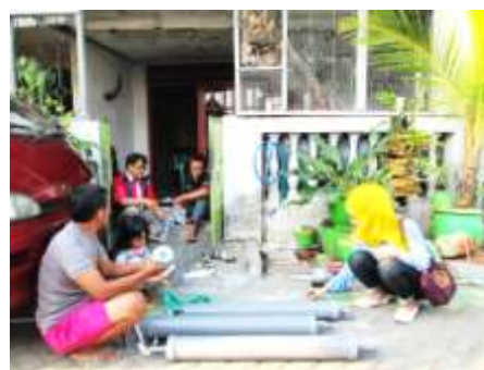
Figure 2: Residents are working on a simple WWTP
