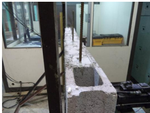
Figure 2. Regular concrete test wall under construction
