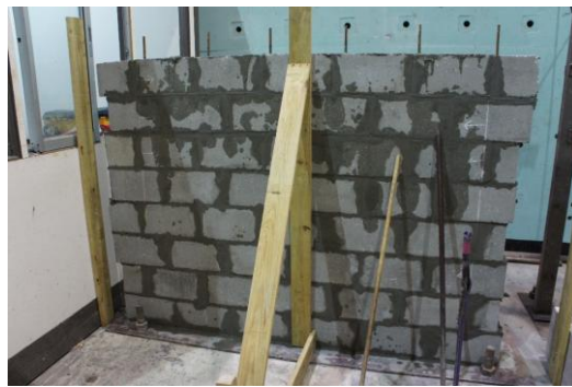
Figure 4. Completed interlocking block wall section with rebar
